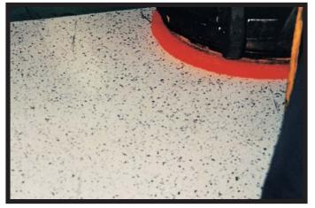
4. The floor was simply scrubbed with 3M<sup>™</sup> Neutral pH Cleaner and a low-speed buffer per 3M maintenance instructions and allowed to dry.
