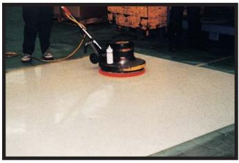
5. The clean floor was then polished with a low-speed buffer. The badly abused floor looks like new and NO WAX OF ANY KIND WAS USED.
